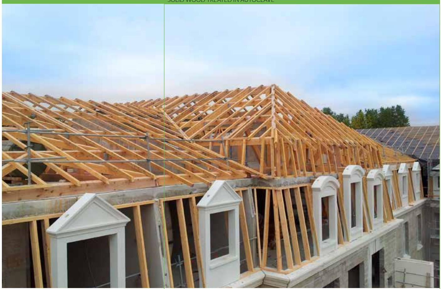
**MADEIRAS LAMELADAS COLADAS TRATADAS EM AUTOCLAVE** BOIS LAMELLÉ-COLLÉ TRAITÉ EN AUTOCLAVE
